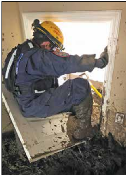
Alhambra Firefighter crawls through the window of a house filled with mud.
